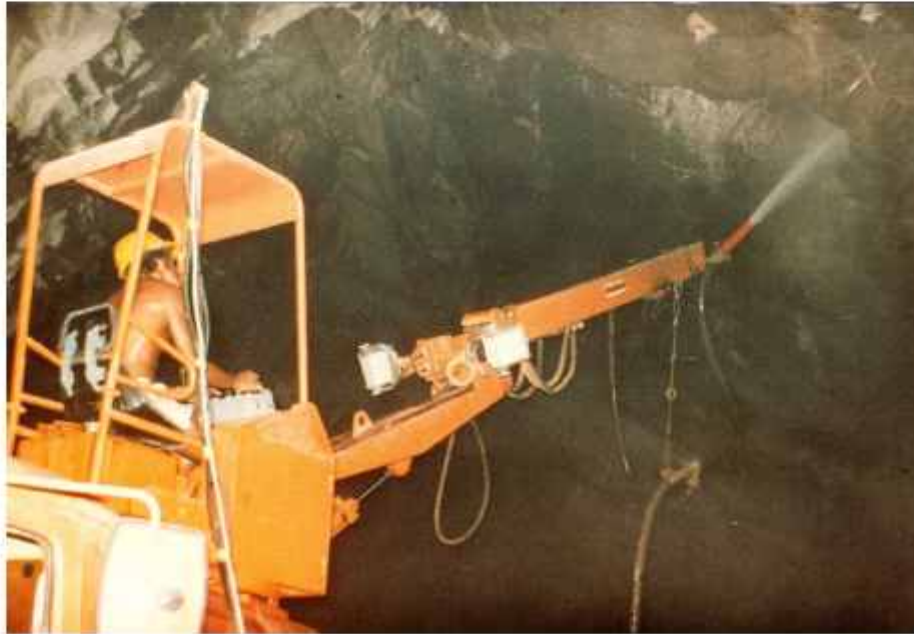
Figure 9: A truck mounted shotcrete robot being used in a large civil engineering tunnel. Note that the distance between the nozzle and the rock surface is approximately one metre.
